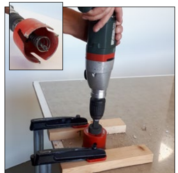
Opening using a hard metal core drill
