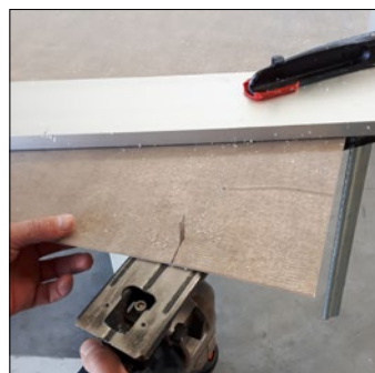
Cutting to length with a jigsaw
